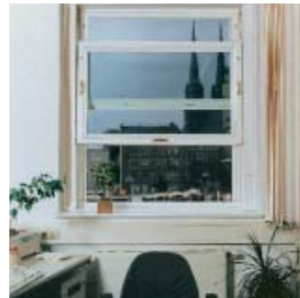
Space-saving can be so elegant: Town Hall, Halle/Saale, Germany.
