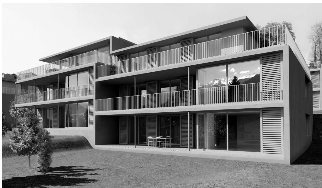
Example stacking 90° to the slide axis: The shutters run in front of the parapet and provide shade on the balcony.
